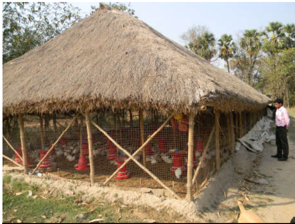
Low cost broiler shed
